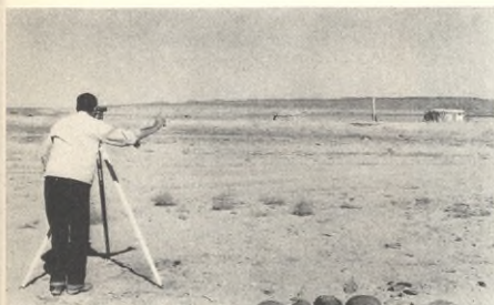
First step in seismic survey at Four Corners is staking out of test area.
