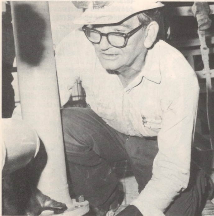
C.J. Bryant, a South pipefitter, prepares to put bolts in a pipe at the ECH stripper.
