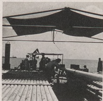
Below, a crew on a special barge lays gathering lines from Shell's underwater wells.
