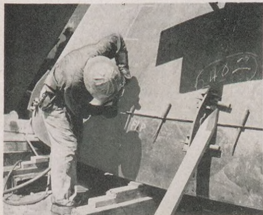
This man is inserting "chucks," or metal clamps which hold metal sections together until the welders come along to make the final joint.
