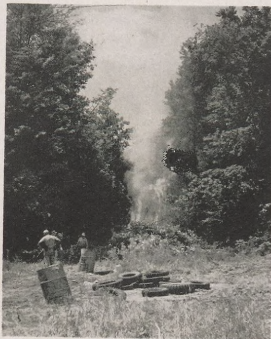
The land along the path of the new products pipe line is generally fairly level. But large oak trees have had to be felled (as at left) and brush burned through forest areas (as above) to clear the right-of-way for bulldozers and other necessary pipe line construction equipment.
