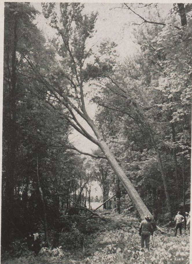
The land along the path of the new products pipe line is generally fairly level. But large oak trees have had to be felled (as at left) and brush burned through forest areas (as above) to clear the right-of-way for bulldozers and other necessary pipe line construction equipment.
