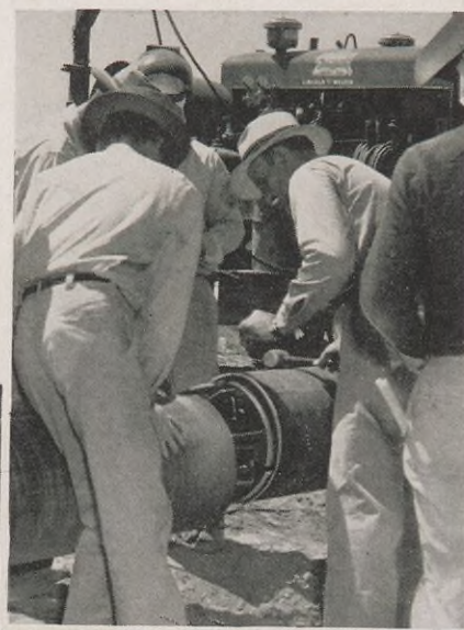
Construction scenes: A beveling machine is used, above, to cut a pipe joint to the proper angle. Below: an inside line-up clamp aligns two joints for the welding shown, left, below.
