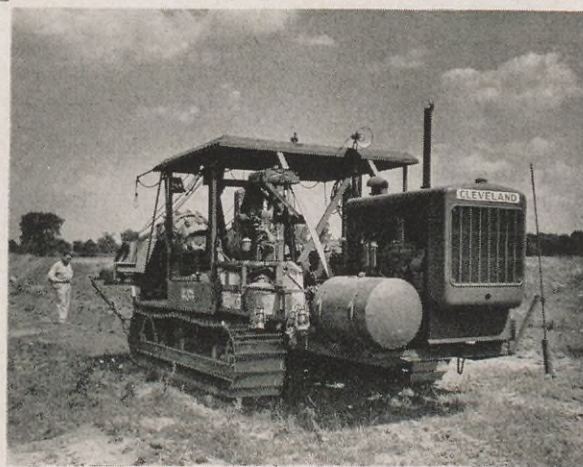
A ditching machine, above, cuts a trench for the pipe along the cleared right-of-way. Before it is laid, the pipe is coated with tar to protect it from the corroding action of the soil. Whitewash is added later, left, to reduce the pipe's absorption of solar heat. In swampy areas, a coating of cement is added to protect the pipe and anchor it firmly in position.
