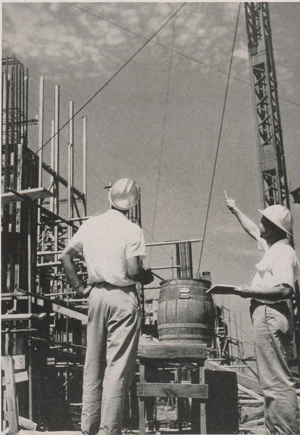
Shell personnel constantly check construction progress as Norco continues to grow. Here, Dwight Pfahler and Earl Crochet look over the forms being erected to facilitate building a concrete column. Steel columns and cross beams are sometimes encased in concrete as a fireproofing measure.
