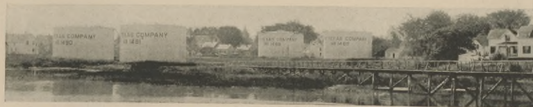
Tank Field—Portland Terminal
