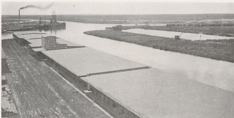
Texaco Overlap Roofing with Asphalt Top Finish, 170,000 square feet, applied to roof of Port Arthur Canal and Dock Company's Warehouse, Port Arthur, Texas
