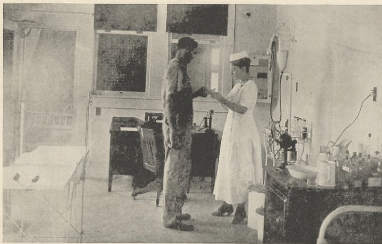
First Aid Room, trained nurse in attendance, Port Arthur Case and Package Plant
