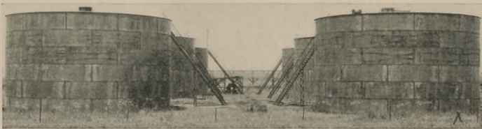
Six 12,000-barrel tanks under construction at West Dallas Works
