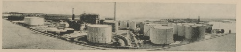
Norfolk Terminal—Asphalt Plant at Left of Center
