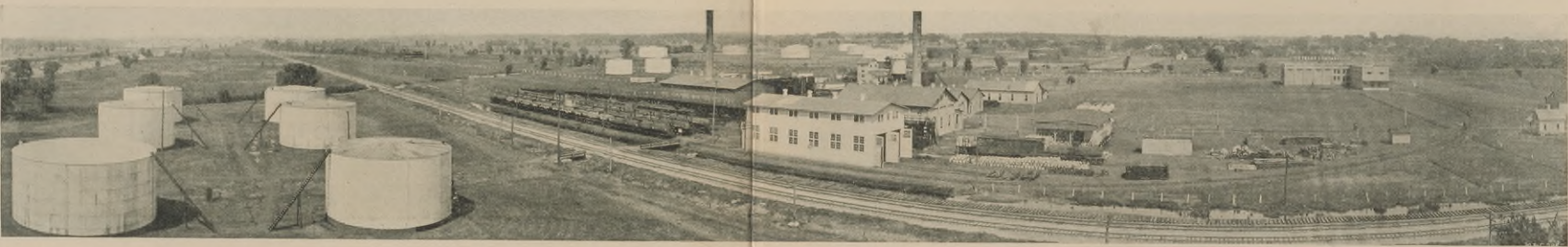
Lockport Works — Looking East
