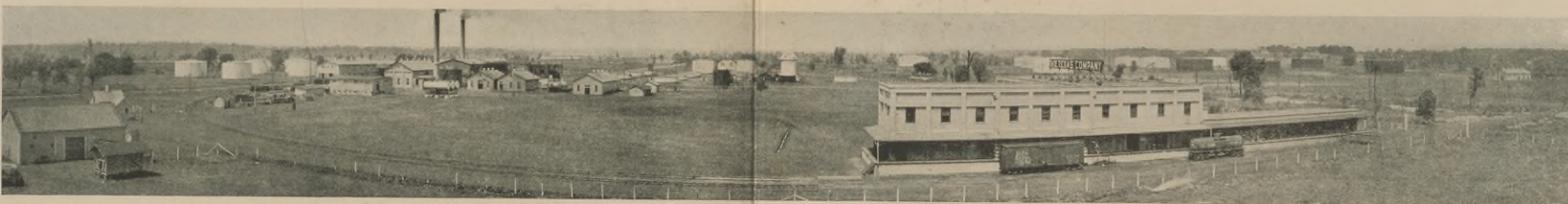
Lockport Works — Looking North
