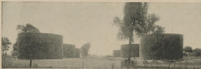
Six 12,000-barrel tanks under construction at West Tulsa Works
