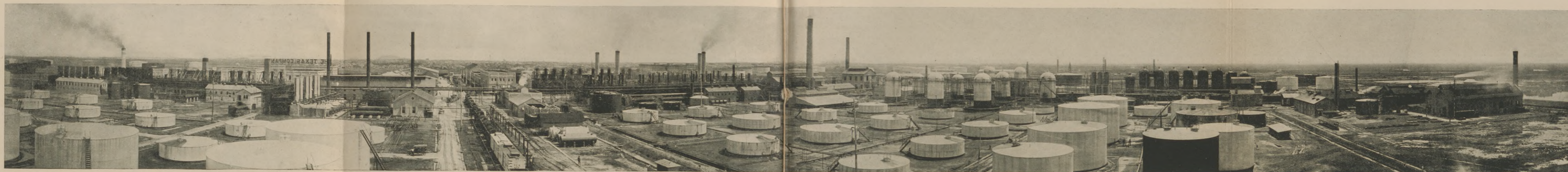
Port Arthur Works — Looking from rear of Plant
