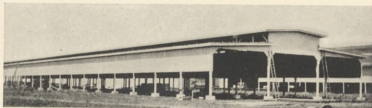
New Cooling Sheds, Port Neches Works
