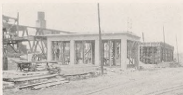
Chicago-Archer Avenue Station in course of construction—Office and Garage
