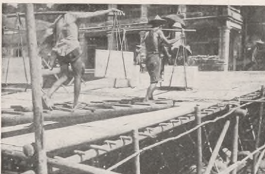
Bamboo Tetty for Discharging Scale Oil—Hong Kong "Scale" is The Texas Company's registered brand in China
