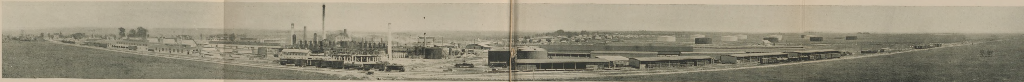
Port Neches Works
