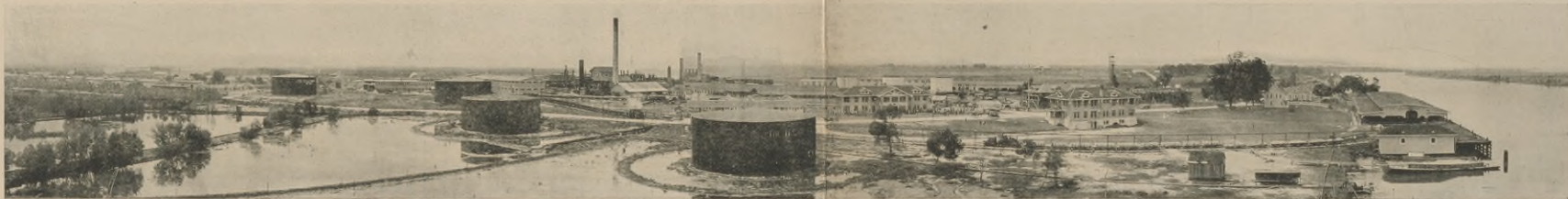
Port Neches Works
