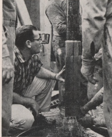
TOP, LEFT: Operations on this deep Shell Oil Company wildcat were brought to a halt when a "fish" consisting of drill collars and bit twisted off in the hole more than 18,000 feet below the surface: TOP, RIGHT: The crew will soon know whether they've caught their fish or not, as the last joints of more than three miles of drill pipe emerge from the hole. BOTTOM, LEFT: This one got away. Shell drilling engineer B. J. Bullard kneels to examine the empty fishing tool, which was supposed to have grasped the fish and hauled it to the surface. It took about 24 hours to run the tool into the hole and back out again. BOTTOM, RIGHT: Bullard checks the grapple which fits inside the fishing tool. Close inspection showed that the grapple's teeth never engaged the fish. On the next trip, however, the fish was caught and successfully removed from the hole.
