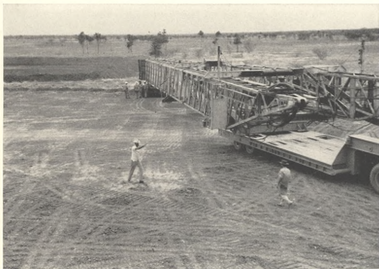
The Las Mercedes concession reminds oilmen of Rio Grande country in West Texas. Here a portable drilling mast is being swung by trailer-truck to a spot in which a rig will be set up. When erected, the mast will stand 137 feet high.
