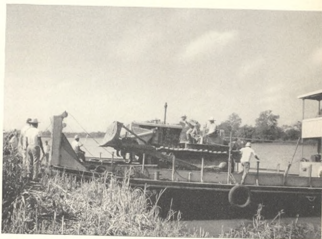
At Tucupita this bulldozer will clear a roadway to well site. Like other equipment, it had to be barged to the field.
