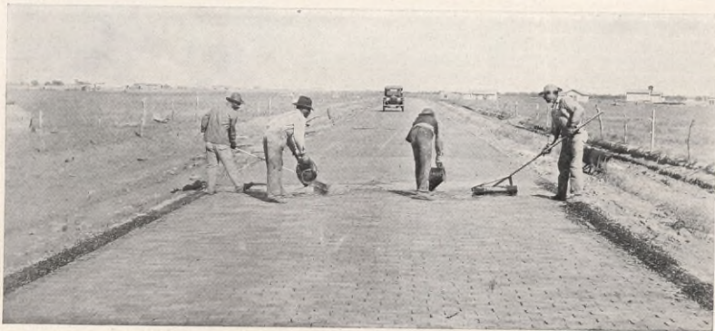
Twenty-one miles of asphalt-filled brick, Eastland County, Texas
