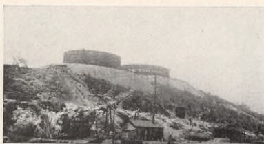
Guayanilla, Porto Rico Station of The Texas Company (P. R.) Inc. New gasoline tank nearly completed
