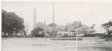
Savannah Sugar Refinery, Savannah, Ga.—Well satisfied with Texaco Crater Compound for gear lubrication
