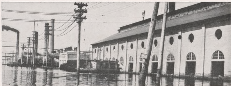
No. 2 Boiler House, August 29, 1915. Note cofferdams in doorways.
