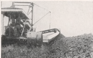
Buckeye Ditcher No. 1 working on levee.
