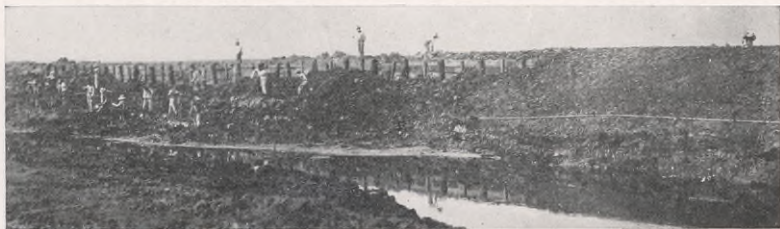
Driving revetment to reinforce levee across a stretch of marshy ground.
