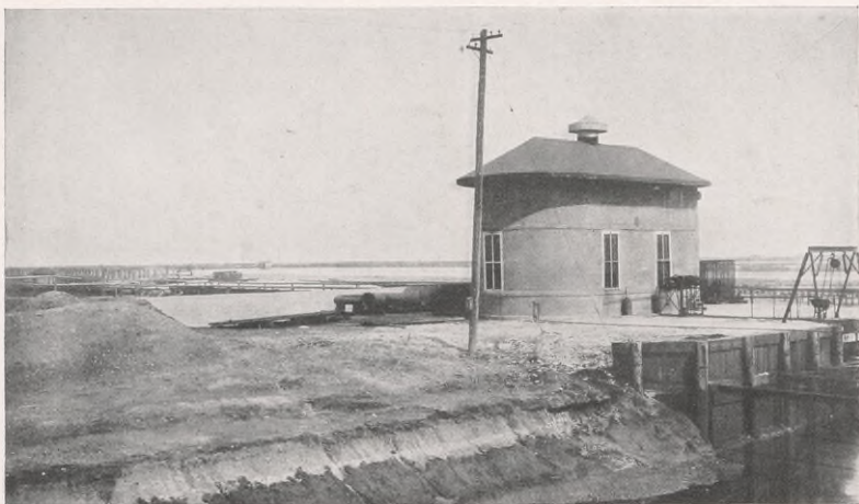
Main Drainage Pumping Plant, two centrifugal pumps, capacity 35 million gallons per day.
