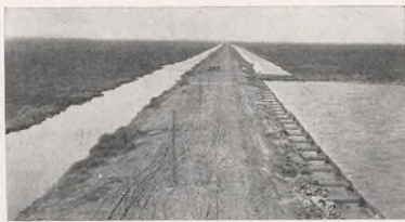
Levee used to elevate main pipe lines above a salty marsh. Area subject to inundation at left. Ditch at right conducts drainage (fresh water) from Port Neches to Port Arthur Works, 8½ miles.
