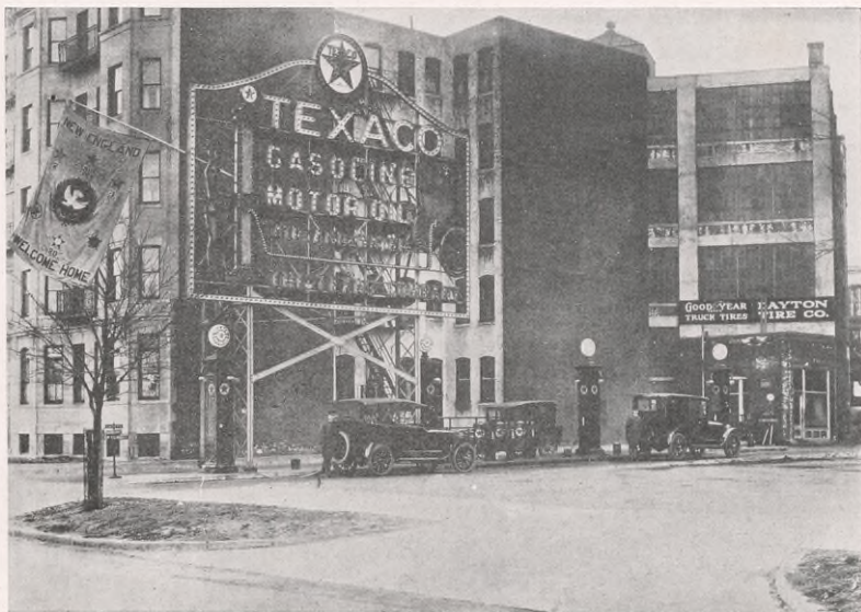
Boston Commonwealth-Beacon St. Filling Station.
