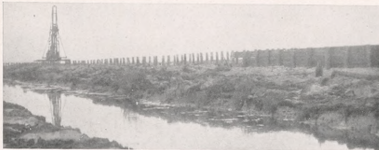
Finishing a reinforced section of the levee.
