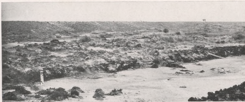
A section of completed levee across marshy ground.
