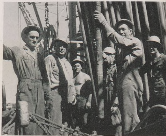
Logging equipment is poised for its descent into the hole at Weeks Island Rig No. 3 as the crew looks on. This rig is drilling the first well on the field's eastern flank.
