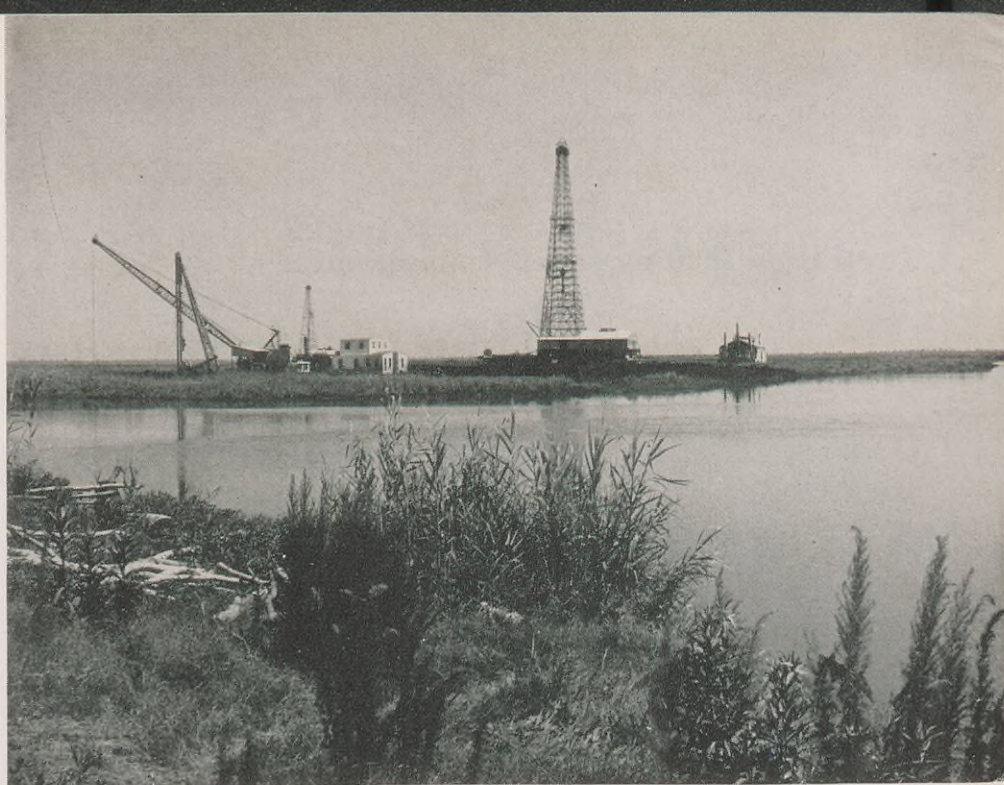
Rig No. 7 at Weeks Island is completing a well as pilings are being driven for the next drilling location. Shell has pioneered advances in deep drilling techniques in the area and records in drilling time, depth and production have continually been made and broken. Shell's gross share of oil from the Weeks Island field averaged more than 24,000 barrels per day for June, 1952.
