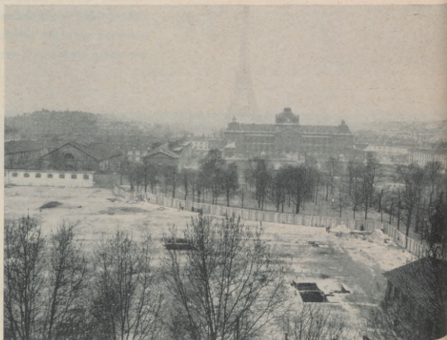
New headquarters for UNESCO are being constructed on the Place de Fontenoy in Paris, with sight of the Military School of Paris and the Eiffel Tower. The building will be seven stories high with a housing capacity for 1500, a parking lot for 150 cars, an additional underground garage, and a conference room for 1500. It is expected to be completed within the first six months of 1957.
