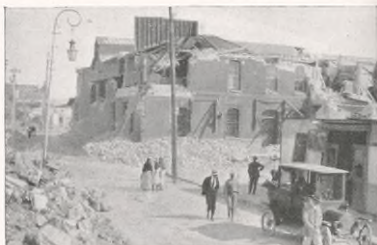
Electric Light Plant
