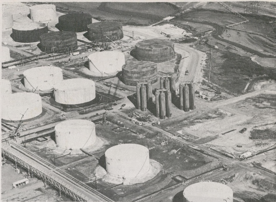
FOR THE FIRST TIME at the Refinery, high pressure propane storage tanks have been installed vertically.
