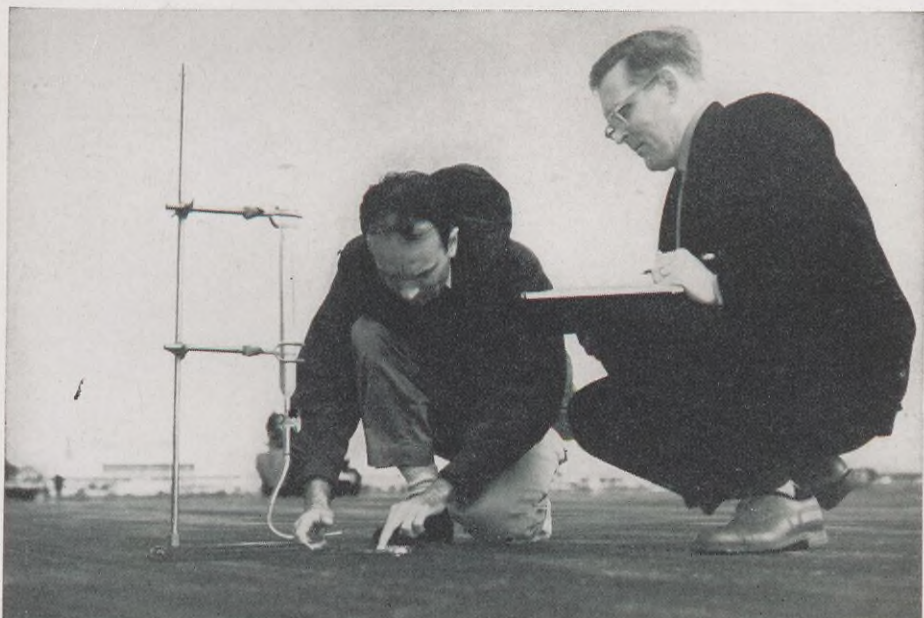
Testing the pavement are Laboratory Assistants A. B. Cox, left, of Emeryville's Bitumen Department and Chemist L. R. Roberts on assignment from Shell Oil's Martinez Research Laboratory to Shell Development. The test determines the pavement's permeability (the amount of fluid it will absorb). The tube contains water and detergent. The new product passed the test.
