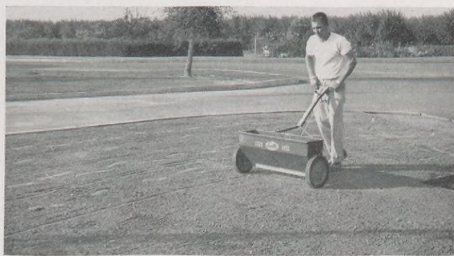
4... Apply quality seed mixture with a spreader
