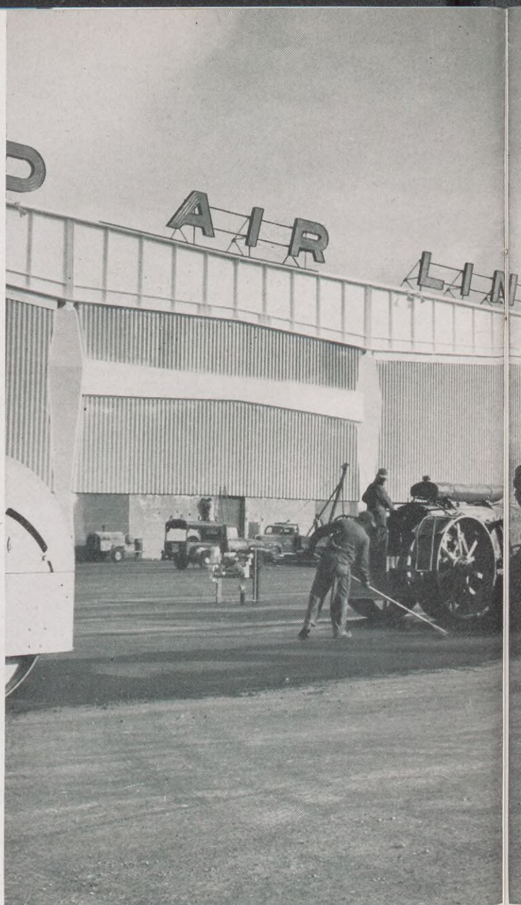
Paving operations move ahead to cover 3½ acres of the jet aircraft parking apron in front of the United Air Lines hangar at San Francisco's International Airport. Because the asphalt must
