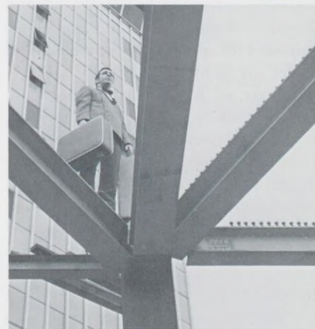
PRE-VIEW —Dave Paulon, Anchorage Westward Executive Assistant Manager, gets a pre-view of the hotel's tower construction from his precarious steel framework perch. Wearing a Bellman's uniform and carrying a suitcase, Dave attempts to visualize what the 22-story addition will look like when completed late this year.
