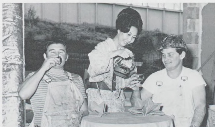
TEA FOR TWO —Miyako Construction workers after a busy morning at the hotel site, pause for a tea-break and are graciously served by diminutive Miyoko-san, a Miyako Waitress. The San Francisco Japanese styled hotel is now involved in an expansion program that, when completed by June 1971, will include a new banquet room, (the Imperial Room) a second smaller banquet room, enlargement of the present Garden Bar and Spring Room, and the addition of seven deluxe suites.
