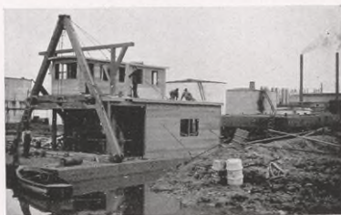
Dredge No. 4—Picture taken while the house was being built on it, and while the steel hull for Dredge No. 5 was on the ways ready for launching.
