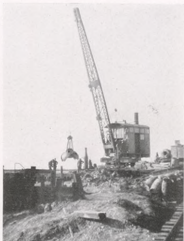
Locomotive Crane and Clam Shell Bucket excavating the pits enclosed with steel sheet piles.
