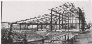
Pump House No. 1—Structural steel frame work.
