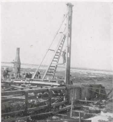
Pile Driver No. 2 constructing revetments on marshy ground for reservoir levees.
