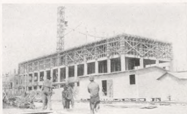
Concreting roof of new Can Factory.
