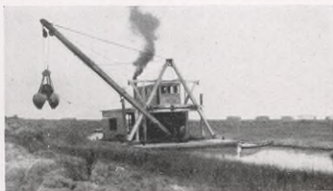
Dredge No. 2, built on a steel hull 30' wide by 50' long; equipped with boom 64' long, hoisting engine, and a 21 cubic feet clam shell bucket. These dredges are of very shallow draft and can be floated almost anywhere. The regular crew on each consists of three men.
