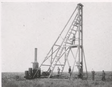
Pile Driver No. 1 driving piles in marsh for 55,000-bbl. tank foundation. Several thousand piles, 24' to 30' long, were driven by these two pile drivers. Both were constructed at the Works.
