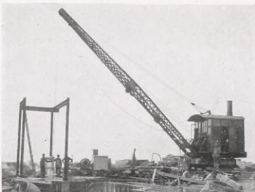
Locomotive Crane lowering pump parts into a pit. The two pumps will have a combined capacity of 35,000,000 gallons for a 24 hour day.
