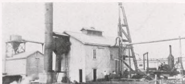
Original Shook Mill Boiler House at Port Arthur Terminal, which was equipped with two 175 h. p. boilers. This plant has recently been increased by adding one 364 h. p. boiler, and the old building has been replaced by a new building.
