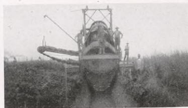
Rear View of Ditcher No. 1, showing ditch 6' wide at top and 6' deep. Operates with crew of three men, handles about 67 cu. yds. per hour.
