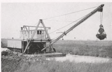
Dredge No. 3; same size and equipment. Each dredge handles about 650 cubic yards in eight hours. Reservoirs and floor protection levees to be constructed in 1916 involve about 475,000 cu. yds. Every dredge is being operated 24 hours a day.
