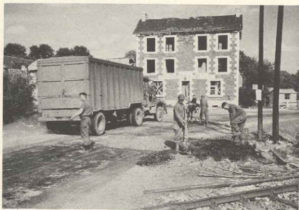
It looks like asphalt. With it, Army Engineers repair a street
