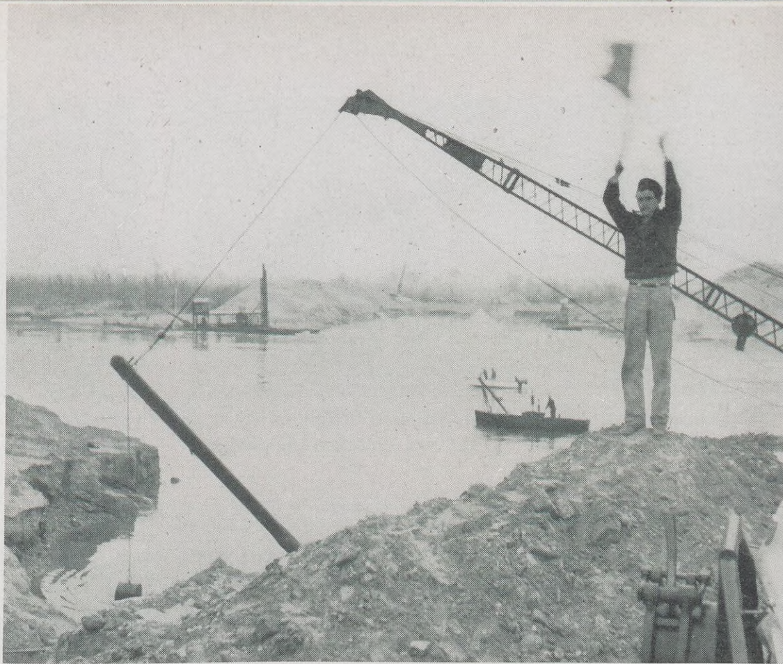
A flagman gives signal instructions as pipe is pulled across the Colorado River near Needles, Calif. The pipe now rests in a ditch on the river's bottom.
