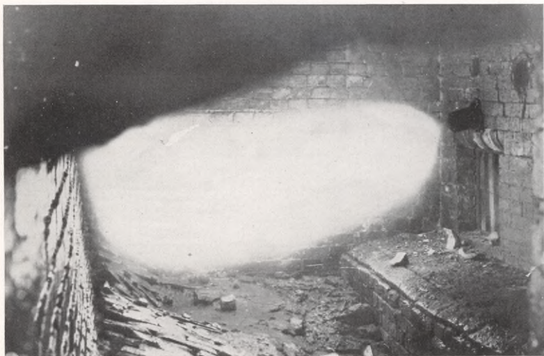
Photograph of flame from oil fuel burner in boiler furnace.—The dark area is shadow, not smoke
