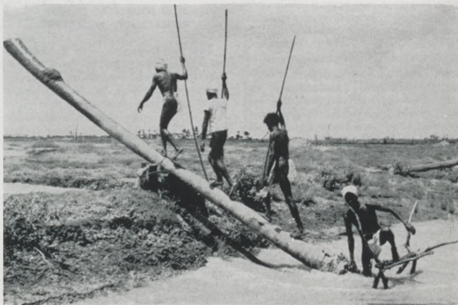
WIDE WORLD PHOTO Peasants in the Godavri Delta area of Madras State in India tread back and forth along the hollow palmyra log to see-saw water through it from the ditch at right for irrigation of a rice paddy. They balance themselves with their long poles and spend hours at each waterpoint, pitting perseverance against the fierce sun. Atomic energy may power irrigation systems in the future.
