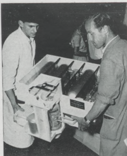
WIDE WORLD PHOTO A Swiss contribution to the atomic display at the Palace of Nations was this scale model of the Babcock and Wilcox "Nuclear Steam Generator." Consolidated Edison Company, of New York, plans to set up this type of generator for their 250,000 K.W. nuclear steam plant at Indian Point, N. Y.
