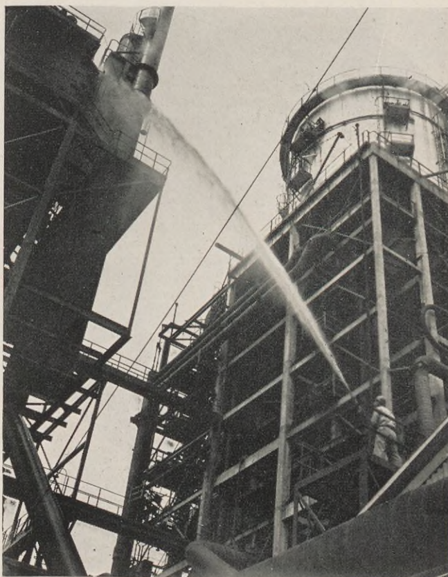
Turret nozzle at catalytic cracking plant. Top of the stream is 200 feet above ground level.
