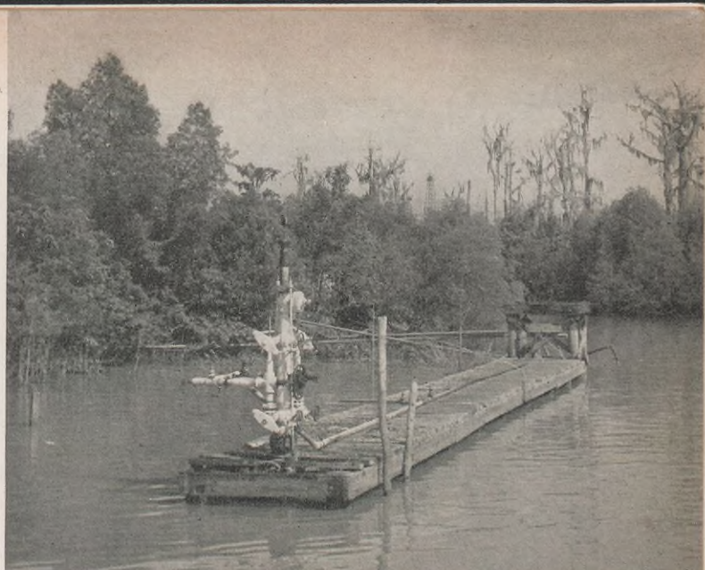
A completed well after the derrick has been moved out
