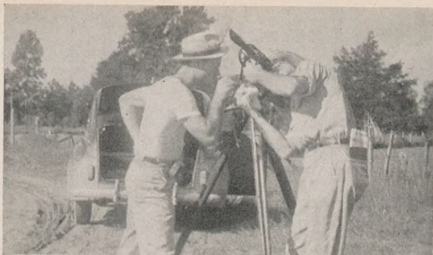
Surveyors making a solar observation to determine directions.
