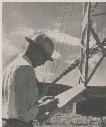
This suspension bridge was built to carry a natural gas pipe line supplying the Jumping Pound Gas and Sulfur Plant in Alberta.
