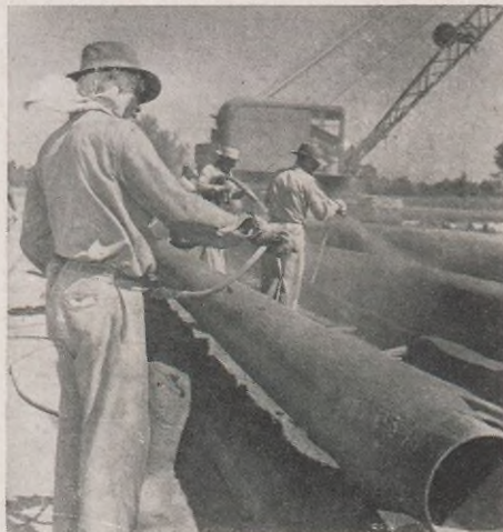
The products pipe line from the Norco Refinery to Baton Rouge goes through swamplands and marshy soil along part of its 65-mile length. A cement coating, such as workmen are applying here, gives pipe greater weight and resistance to corrosion.
