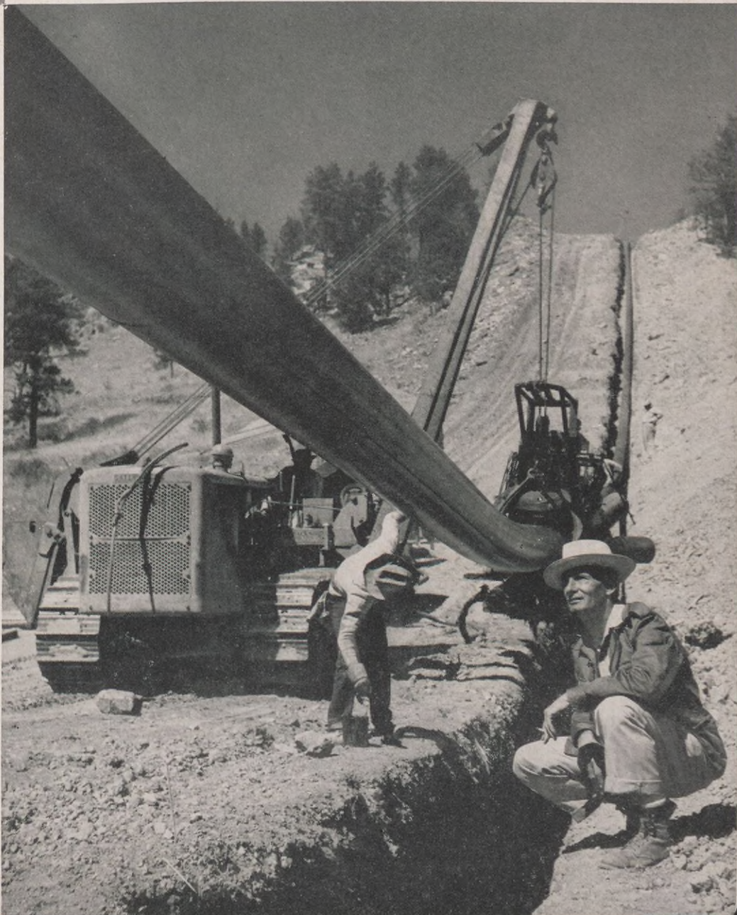
The Butte Pipe Line travels over hills and across rivers and rises from 2,000 to 4,300 feet above sea level to carry crude oil from Montana and Wyoming fields. Here a Shell Pipe Line inspector examines the primer coat on the line before it is wrapped.
