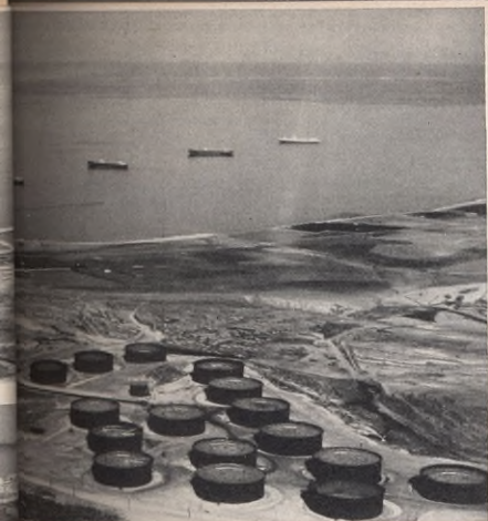
END OF THE LINE —Tapline's Sidon Terminal tank farm, overlooking the Mediterranean Sea, stores crude oil after journey from Saudi Arabian oil fields. Tankers come offshore and are loaded by gravity from these tanks. Shown above are the first four tankers that were loaded
