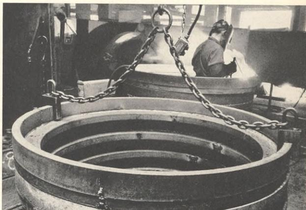
*Heavy sections of cast steel are arc-welded together to produce massive road rollers that pound unruly earth into smooth stretches that become superhighways. Steel stock used in roller production runs as thick as three inches.*
