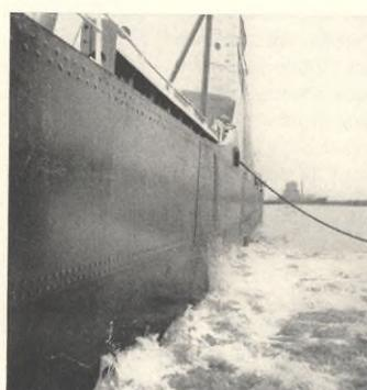
*From the stern of the tug Havoline, a nimble seaman tosses a heaving line to the loaded California. This is a light line, used to haul the heavier towing hawser aboard. With its cargo, crew, and machinery and equipment checked the California is ready to up-anchor and shove off. At near left, wash from the Havoline's screw beats at the tanker's hull as the 565-foot ship swings into the channel.*
