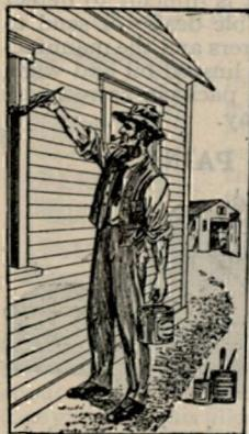
**THE WEATHER.** A dry day should be selected for painting if in any way convenient, however, paint should not be applied when the thermometer registers below 50 degrees, as good painting cannot be done when the paint is chilled. This thickens it and makes it impossible to do a good job, as the coat will be heavy and streaked.
