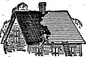
or warp and will double the life of same. Get an open vessel, pour in the stain, then dip the shingles in the stain and immediately take out, lay aside and proceed with the next until all of the shingles have been dipped. This can be done rapidly and several hundred shingles can be dipped in a short time.
