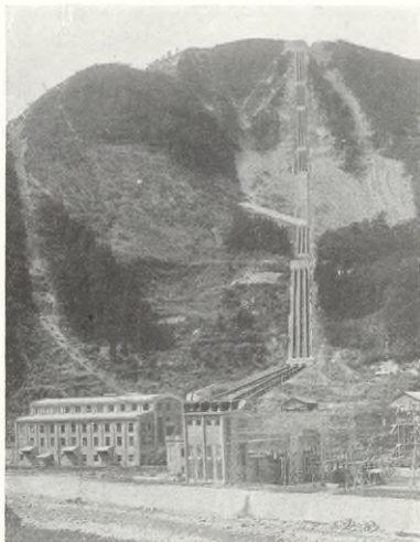
Nakatsugawa No. 1 Generating Station of the Shinyetsu Hydro-Electric Power Company. This station operates under the highest head of any hydro-electric plant in Japan.
