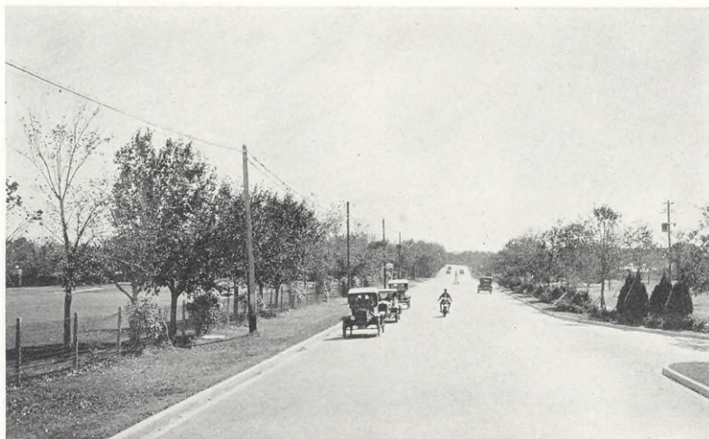
Oak Lawn Avenue is one of many streets in Dallas, Texas, which have been paved with Texaco asphalt
