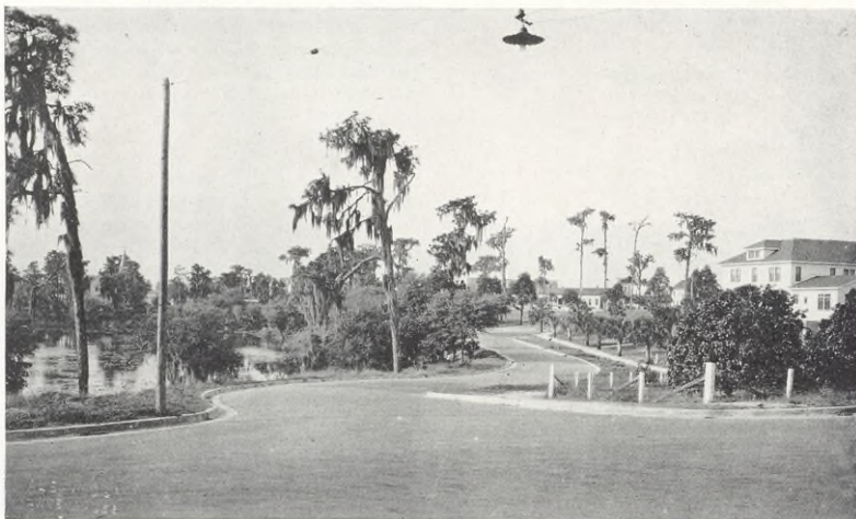
Lake Wales, Florida A Texaco asphalt pavement in most attractive surroundings.
