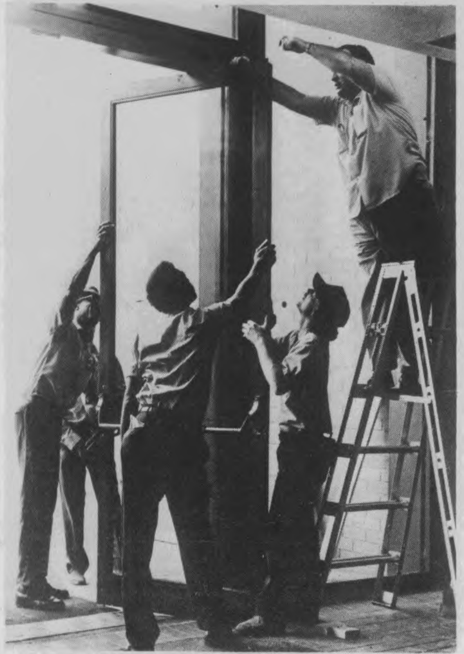
GOT ANY HANGUPS? UH maintenance men hang a new door in the Engineering Bldg. to replace its shattered predecessor.
