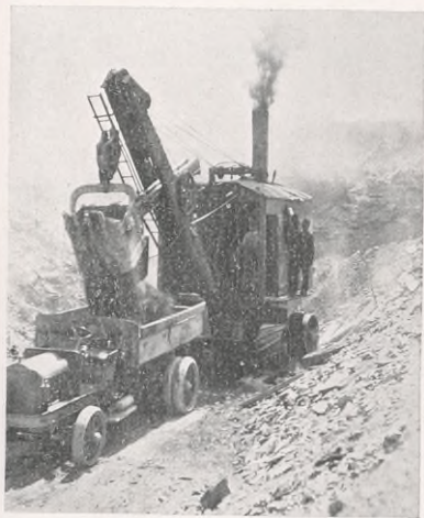
Steam Shovel of the R. C. Storrie Co. at work on a ditch—The cut to be 10 to 40 feet deep when completed—Mr. A. G. Adams, Chief Steam Shovel Engineer, standing in the door of the Steam Shovel—See Mr. Adams's letter
