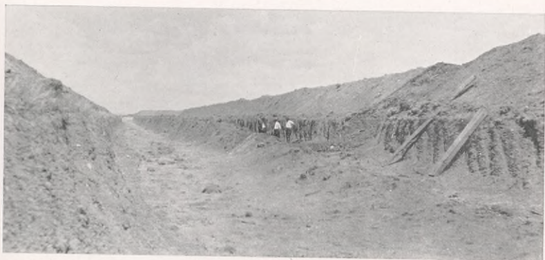
Completed section of a 20-mile ditch of the Storrie Irrigation Works on the Mesa east of Las Vegas, N. M.
