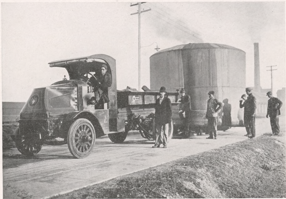
Since the advent of the new trucks at Port Arthur Works many efficiencies have been introduced — Formerly a tank such as this would have been moved by a gang of men or by a team pulling on a fall line — The truck not only pulls the tank along as fast as rollers can be set under it but also carries all the extra blocks and tackle and jacks necessary for the job
