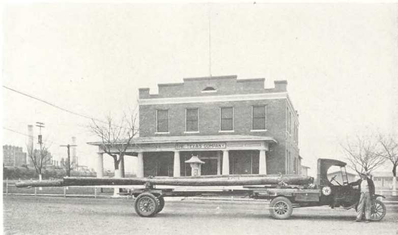
Ready to start for repair job on Tel. & Tel. pole line
