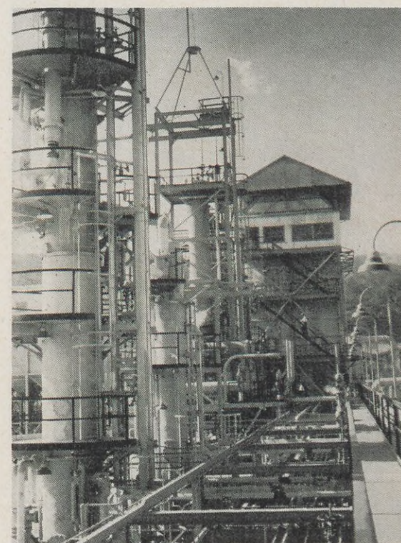
At the end of the catwalk above is the "prill" tower where liquid urea is changed into small spherical particles or prills.
