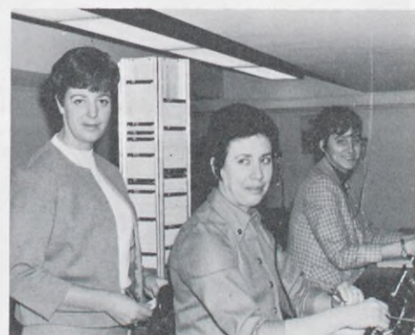
At the switchboard are Chief Operator, Helen Haggart with Operators Fernando Mastro and Cecile Lacelle.
