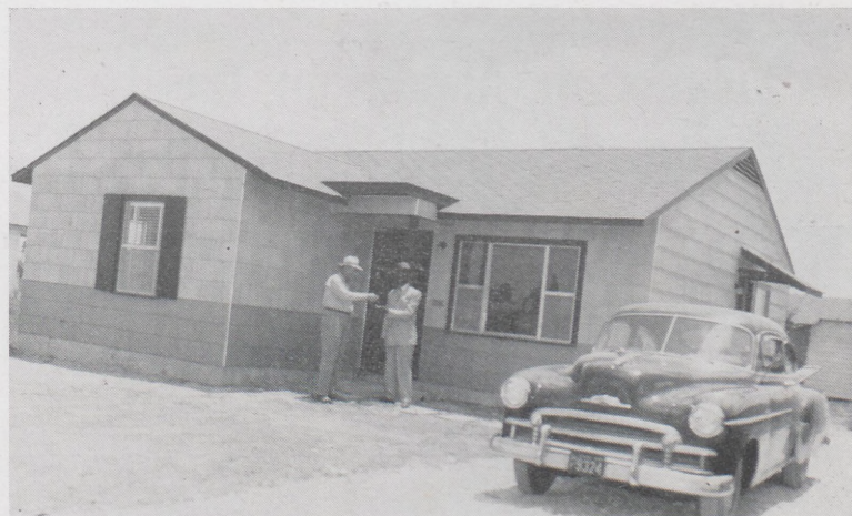
Receiving the keys to his new home is F. J. Lewis (right) of the Labor Department. J. C. McClaran, General Contractor for the job makes the presentation to the proud new home owner.
