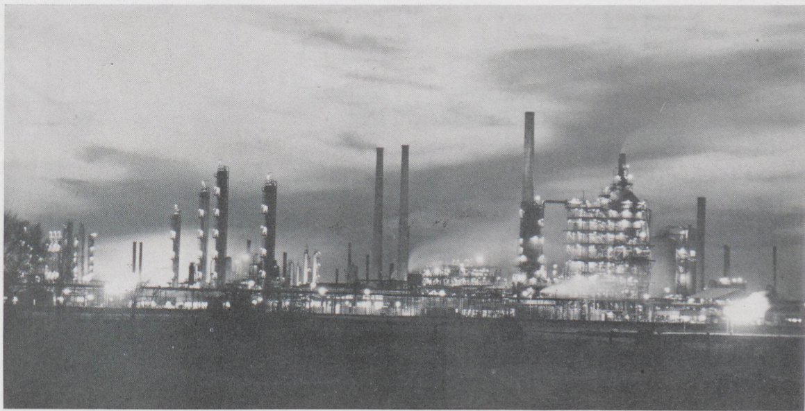
Night view of Houston Refinery's Catalytic Cracker and auxiliary units.
