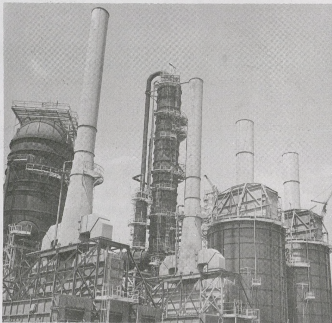
Distilling Unit #2 construction completed.
