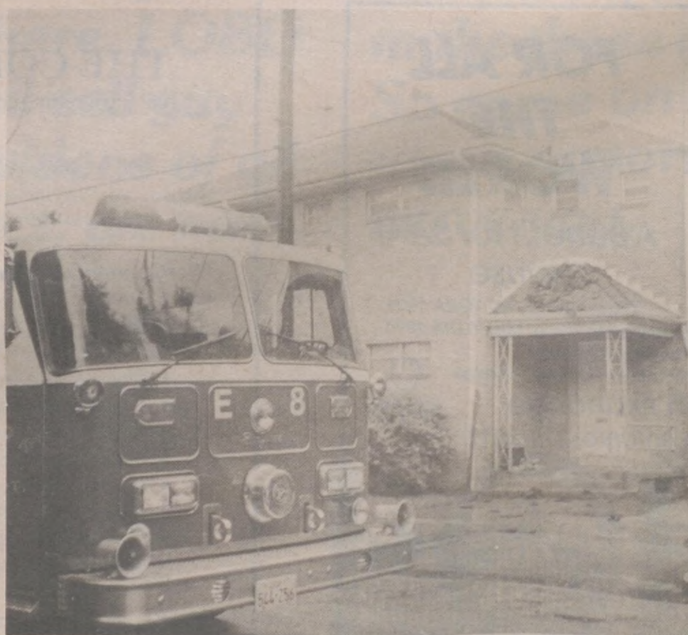
A small fire resulting from lightning striking the Bering Care Center building damaged the roof and electrical wiring, but center activities weren't affected
