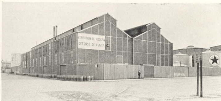
Lubricating Oil Plant at the Antwerp Terminal
