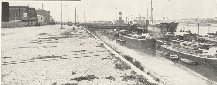
Petroleum Pier at the Antwerp Terminal
