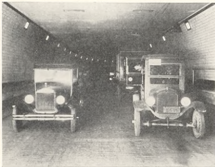
Interior View of the Holland Tunnel
