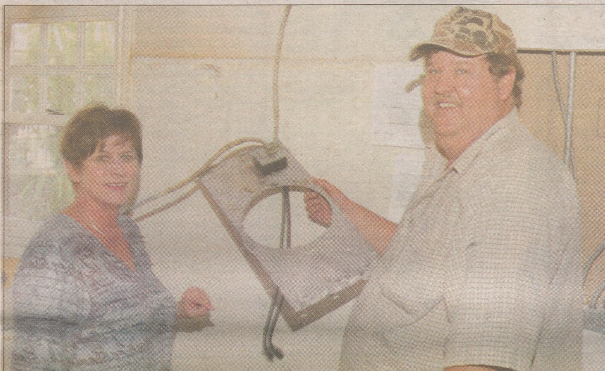
Omega House Director Sandy Stacy and Fred Chalk , facilities manager, stand in the eight-bed hospice's kitchen area, which is currently undergoing renovations.
