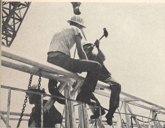
4 A little heavy hammering and the two sections of the mast are truly joined. It only takes a few hours to erect a portable drilling rig.
