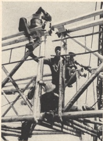
2 Top and bottom portions of tubular-steel mast are slowly pulled together.
