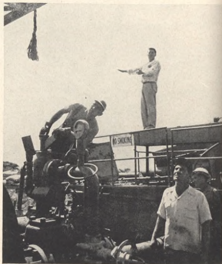
5 Hand signals tell the operator of the hoisting unit what to do next and coordinate the work of those on mast.
