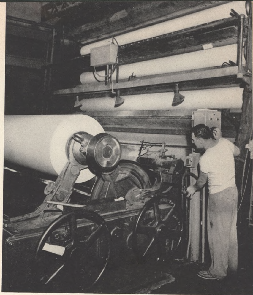
Finished newsprint comes off calender stack. These steel rolls and the dryers are lubricated by recirculating Texaco Paper Machine Oil HD.
