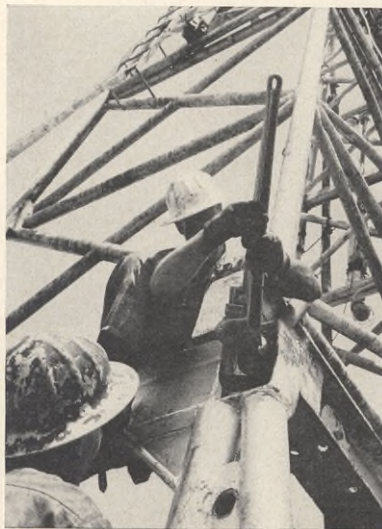
7 As soon as the mast is in a vertical position its hinged legs are secured to the substructure.
