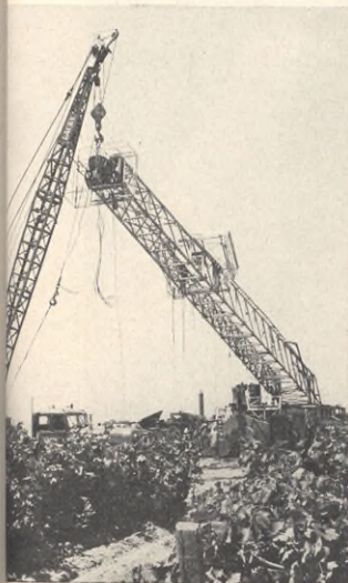
6 This crane starts mast toward erect position. Another will complete job.
