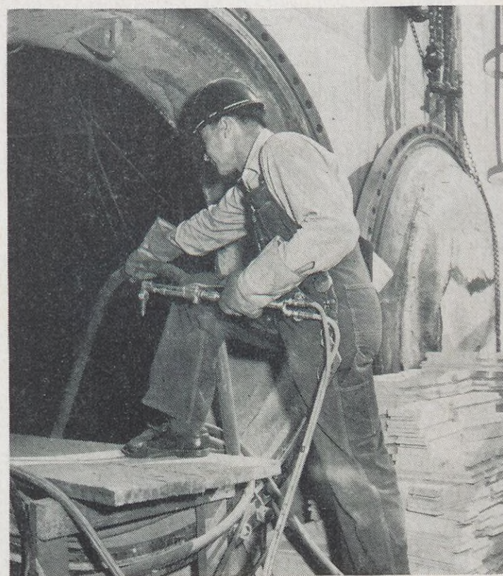
Welder J. L. Elkins enters an access door to a large vessel. The scaffolding inside was erected so the vessel could be cleaned and repaired during the turnaround.
