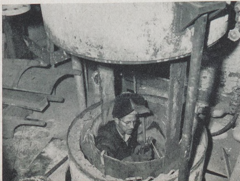
Large sections were cut out of the catalyst stand pipes in the cat cracker so they could be cleaned and repaired. Here Welder L. A. Bapp stands on a platform in the pipe to make repairs.
