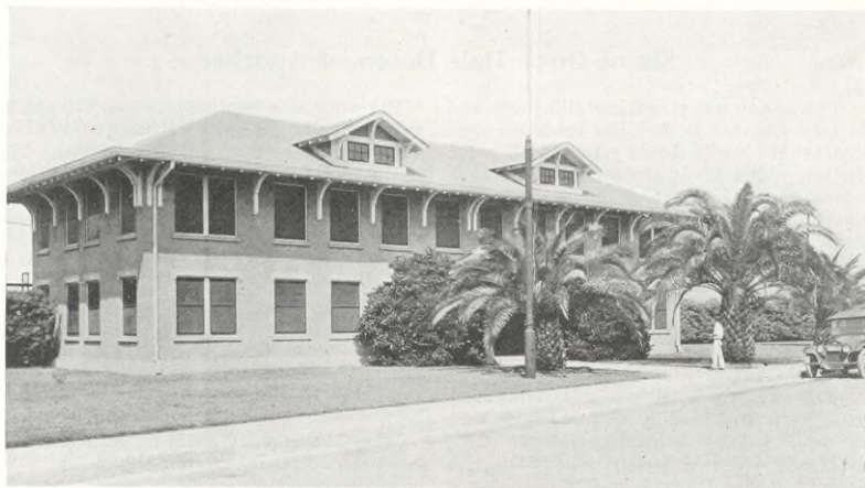
Office Building, Port Neches Works
