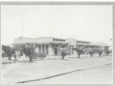
Cafeteria, Port Arthur Works
