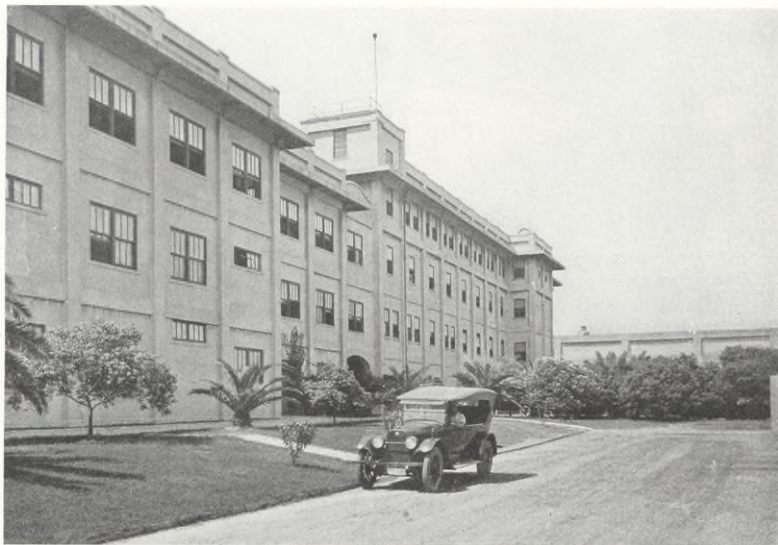
Welfare Building (at left) and Can Factory and Office, Case and Package Div. and Terminal, Port Arthur
