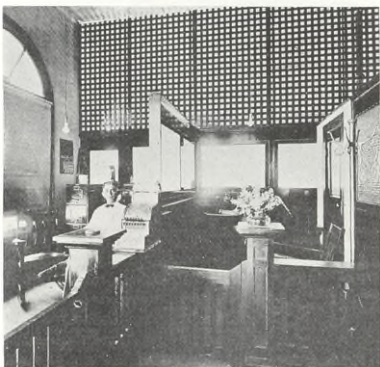
Office in new service station, Hearne, Texas
