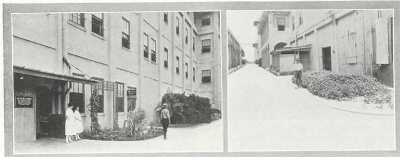
Entrance to Office, Can Factory, and First Aid Room at Port Arthur Terminal and Case and Package Division Flower beds in the heart of the plant
