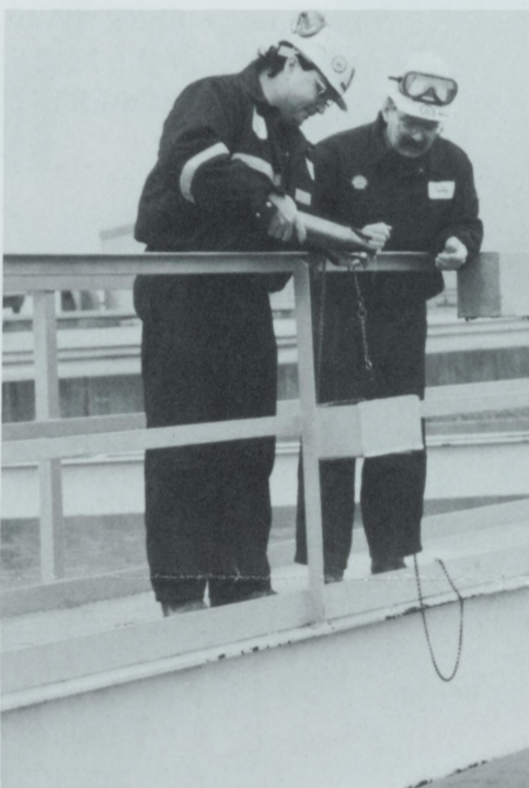
Mike Corron (left) and Terry Harden monitor the water quality of the final clarifiers for clarity.
