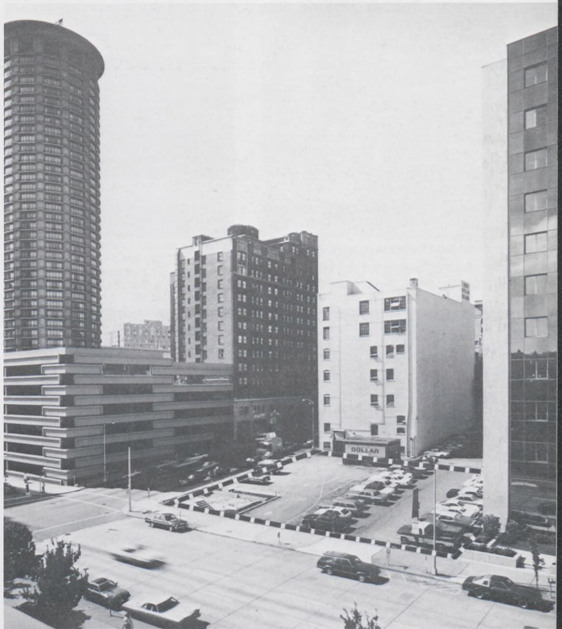
Western International Building site. Tower at left is the Washington Plaza hotel with Benjamin Franklin section to right. White building (center) is the 2000 5th Avenue Building, the proposed parking garage site. A corner of the United Airlines Building is shown at right. (Dotted line indicates position of Western International Bldg.)
