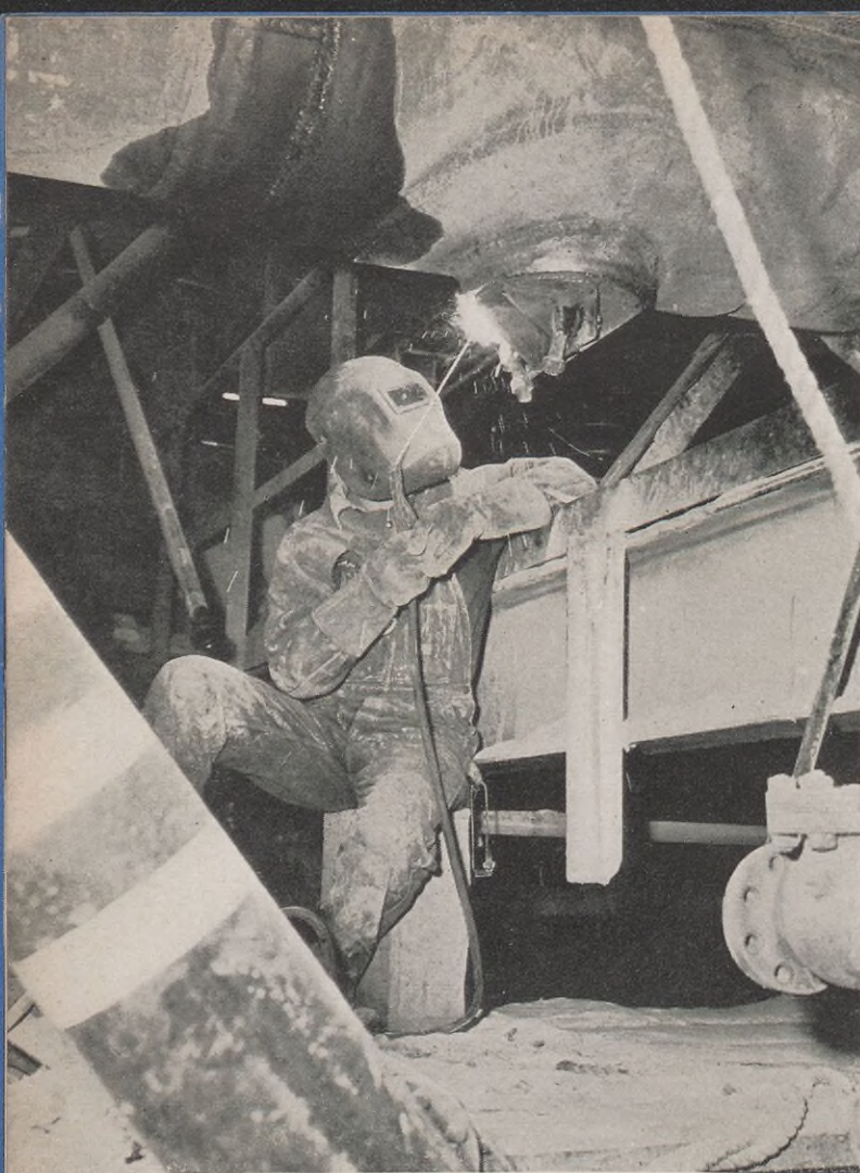
Welders put the finishing touches on one of the "cat" crackers.
