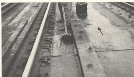
Texaco Rustproof Compound swabbed on railroad bridge decks prevents rust. Arrow shows corrosive brine-drip
