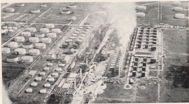
A section of Port Arthur Works showing (in the right-hand part of the picture) 24 Units Holmes-Manley Pressure Stills in operation
