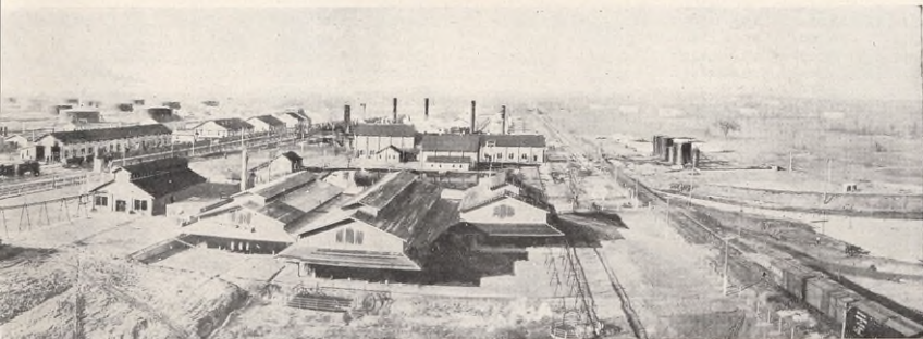
Compression Gasoline Plant and Shed over Pressure Storage Tanks, in right of foreground
