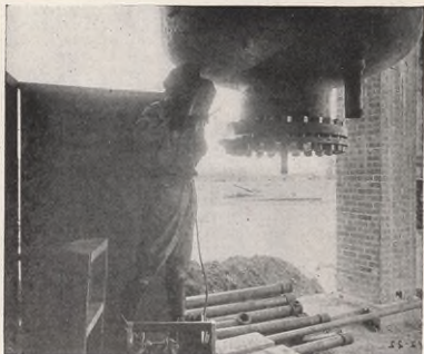
Electrical Welding on bottom of Manway
