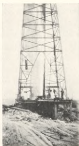
Sulphur Water Well
