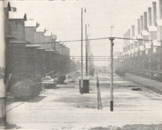
Holmes-Manley Units, Showing Control House, Distillation Columns in Process of Construction and Walkway of Holmes-Manley Vertical Stills
