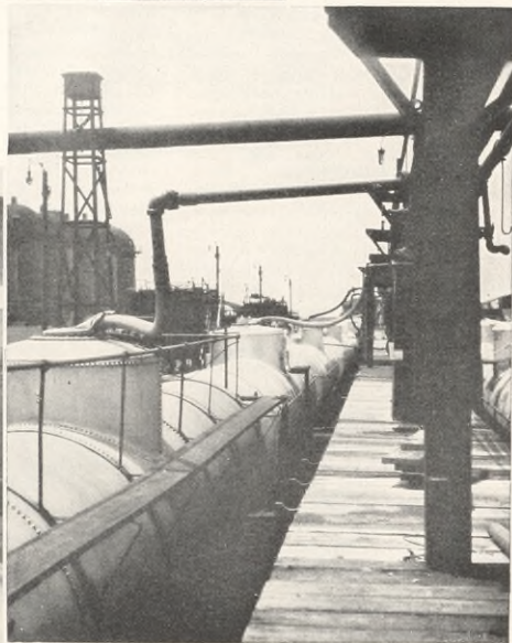
Starting TEXACO Products on their Journey—The Gasoline Loading Rack
