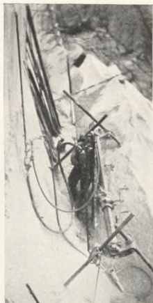
Operating a Drill in a Granite Crevasse
