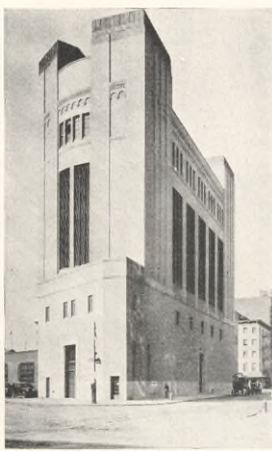
GALLOWAY Ventilating Tower, Holland Tunnel
