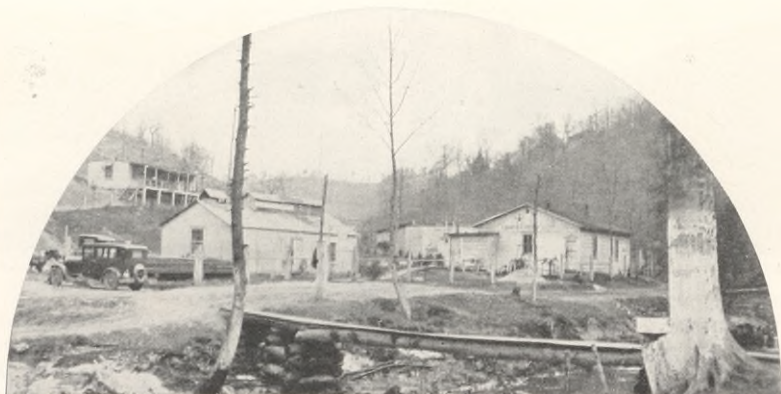
The Texas Company's No. 1 Pump Station, Lee County, Kentucky
