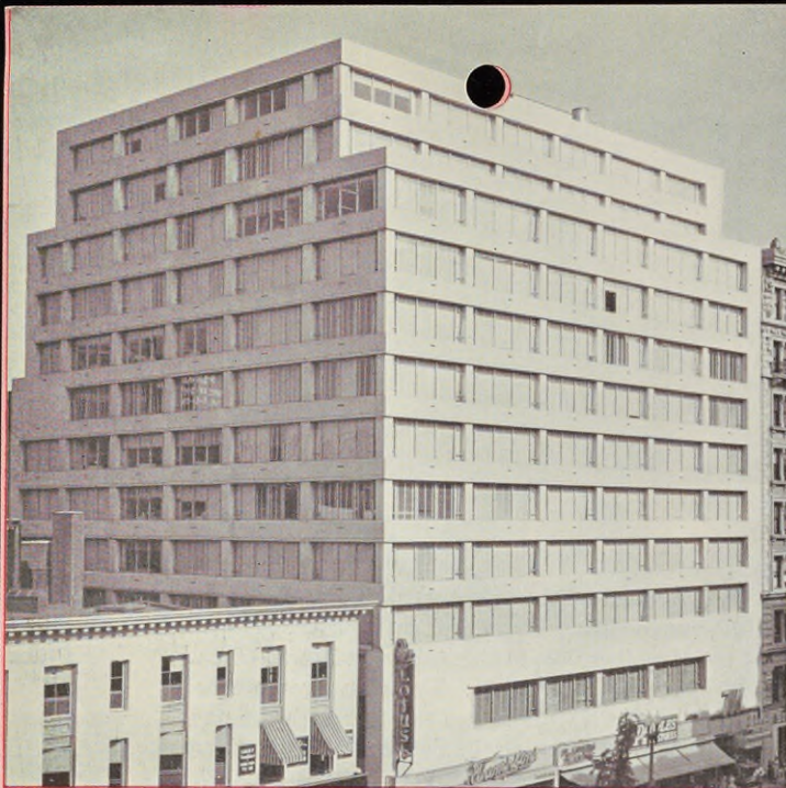
NEWEST ADDITION to the Sheraton family is the Sheraton Building in Washington, D. C. Completed in 1949 it is fully air-conditioned.
