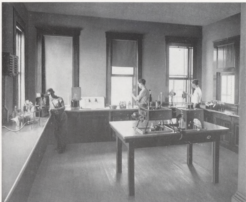
Testing Color, Gravity and Viscosity of Lubricating Oil
