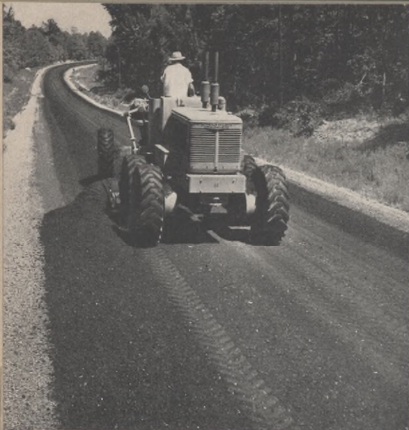
Whatever the volume of traffic, asphalt can provide a surface that is suitable and economical to build and maintain. Here is a farm-to-market road in the process of construction.
