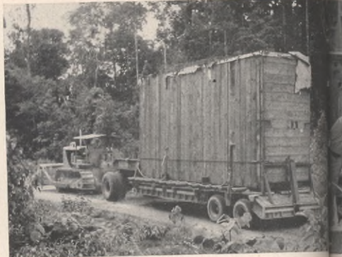
DIFFICULT TASKS constantly confront American oil companies engaged in extracting crude oil from jungle as well as desert regions. Here, in Sumatra, a bulldozer pulls a 50-ton Diesel engine to the Caltex Pacific pump station at the Minas field.
