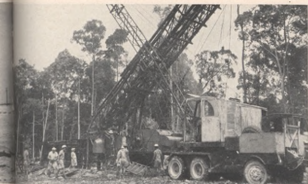
IN THE TROPICAL JUNGLE of Central Sumatra, Americans and native Indonesians combine their efforts in Caltex Pacific's hunt for crude oil. At the Minas field (above) they erect a portable drilling rig.
